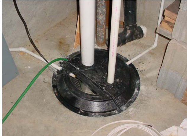
Figure 4-2. Passive sump mitigation system.
