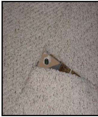
Quarter-sized port to collect sub-slab air
