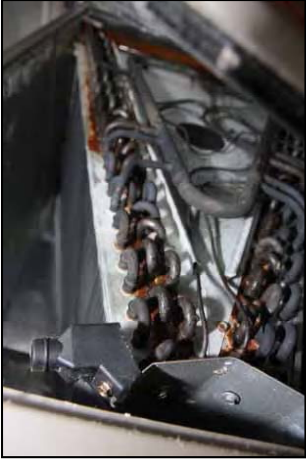
Copper clean outside. Tarnished coils inside. This again is the upstairs AC unit. The downstairs unit is in the garage and not accessible.
